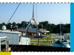
VENTOXAL technology is a submergible technology designed for deep basins (>5m). The different size units allow for sizing small oxygen demands to large oxygen demands.
